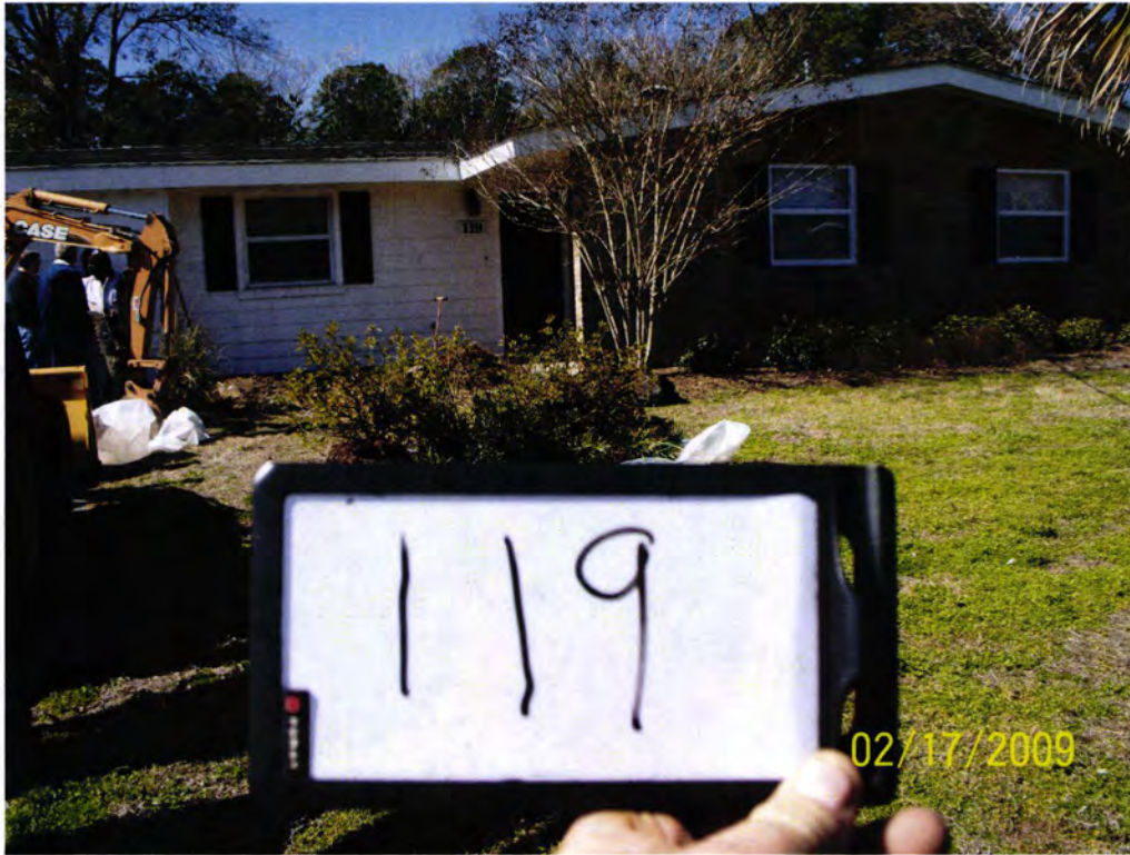
Picture 1: 119 Banyan St. site prior to tank removal.
